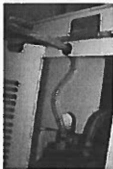
Pump tubing detail, routed from pump, through grommet, to lid.
